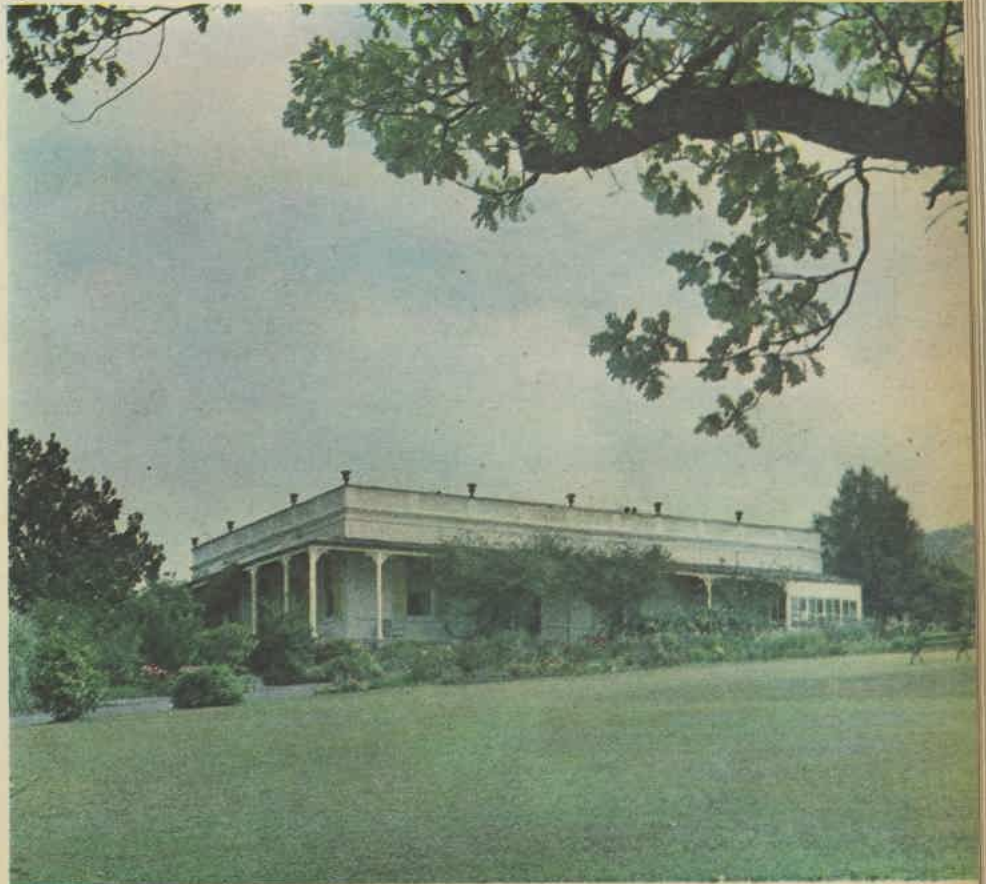
"WINGECARRIBBEE" is a landmark in the district, and its ribbed cast-iron parapet, adorned with ornate urns, can be seen for quite a distance. The house is set on a gentle rise amid lovely gardens. At the back of the house the cemented courtyard, now roofed over, is a workroom-verandah-store.
